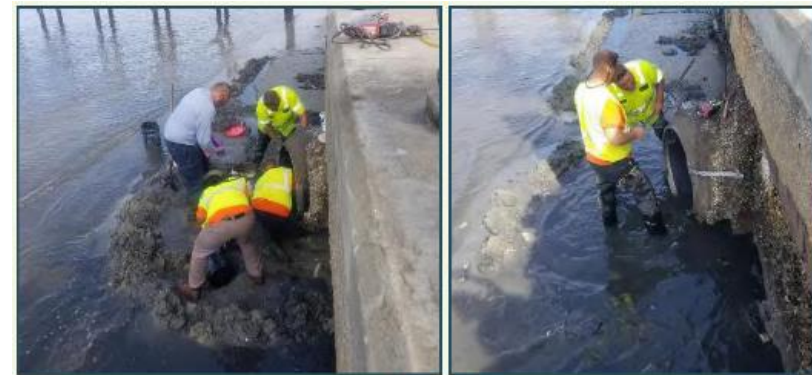
OF-0142 (After): Crew installing valve into outfall pipe
