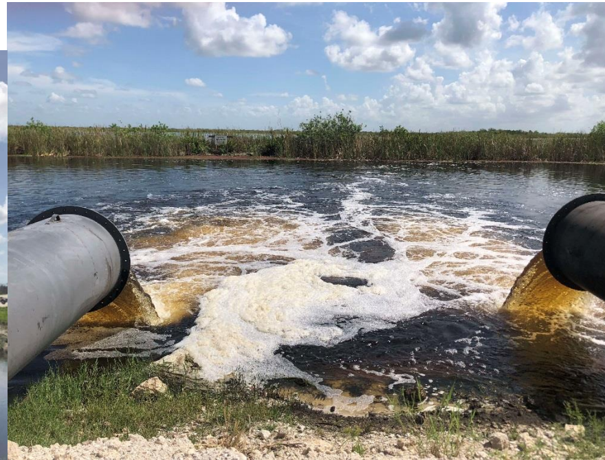
Fig 2: Pumps releasing water from WCA 2 to WCA 1
