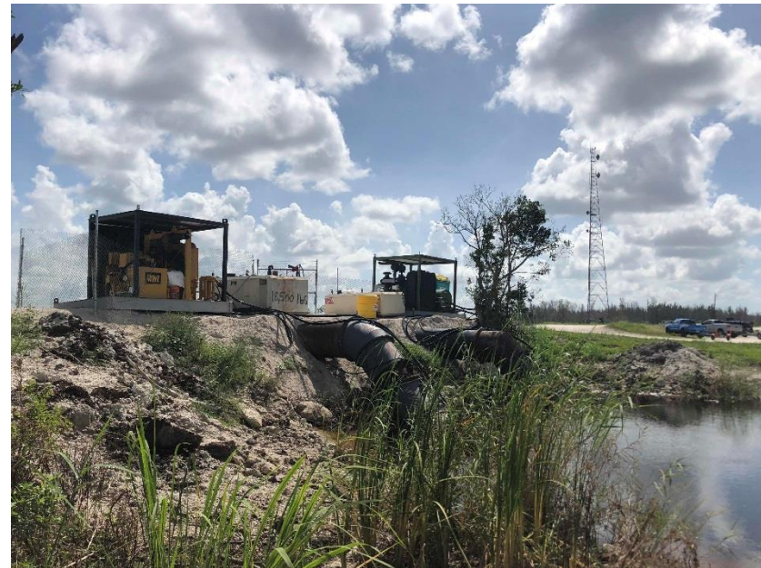
Fig 1: 2- 42" pumps at L-39 moving water through L-39 levee from WCA 2 into WCA 1 near WCA 1 spillway structure
