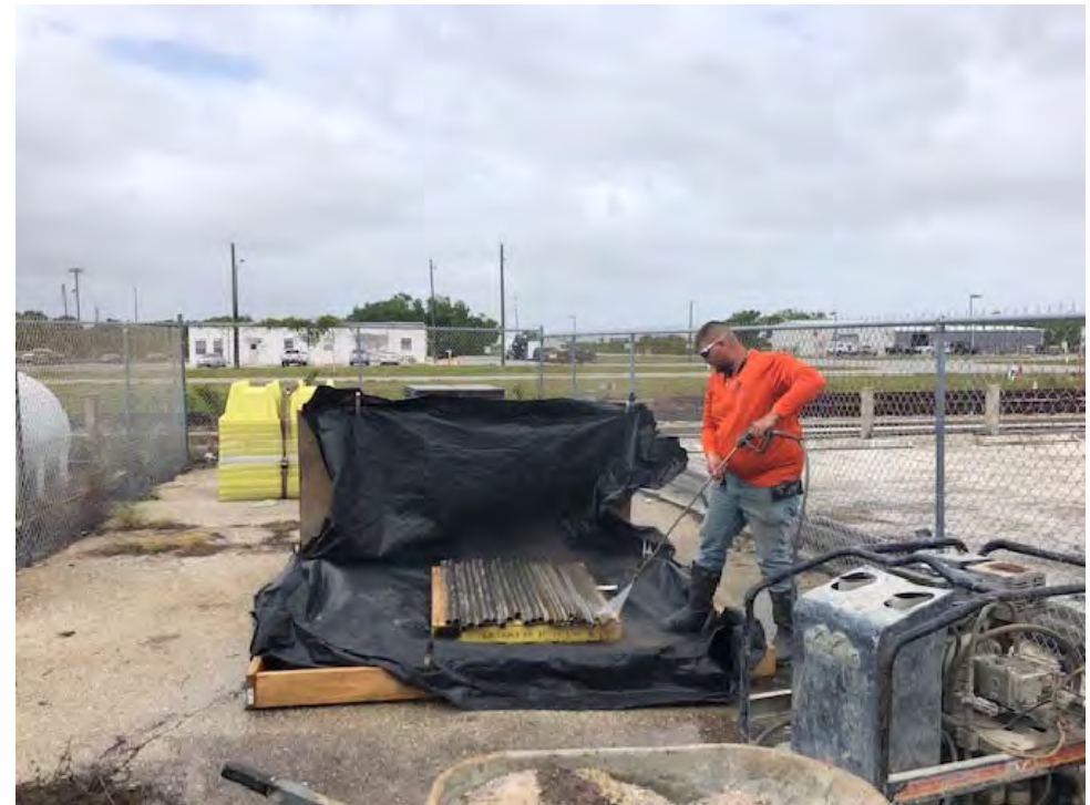
Centrally-located decon pit with pressure washing
